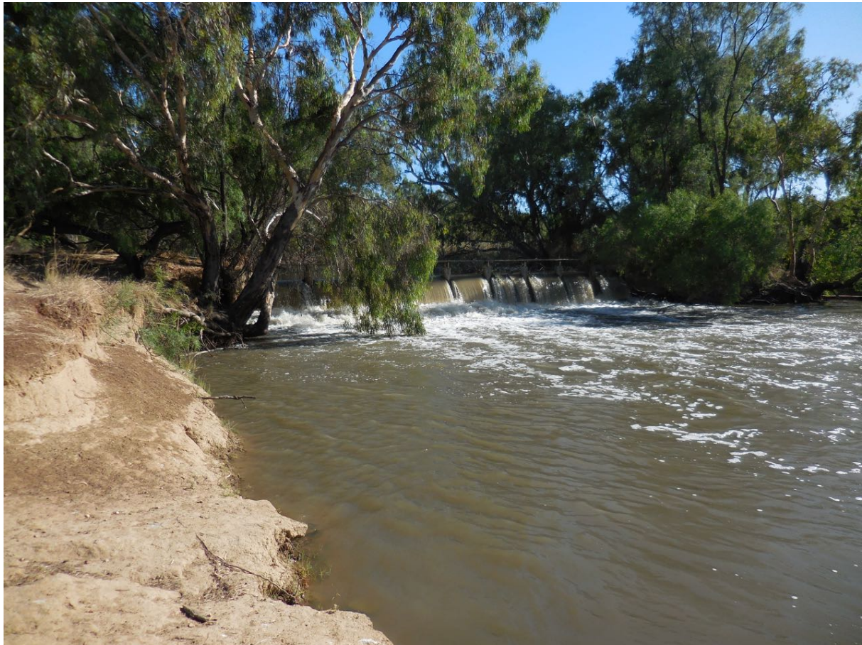
Figure 13. Coonong Weir on Colombo Creek
