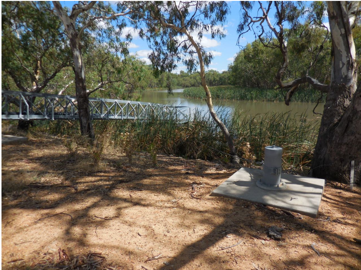
Figure 7. Urana water supply offtake on Colombo Creek
