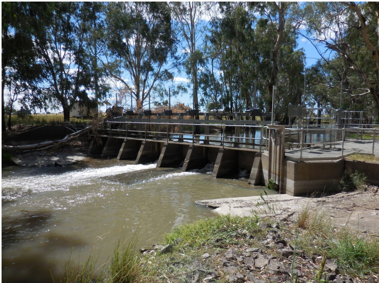
Figure 3. Tarabah Weir and Fishway on the Yanco Creek
