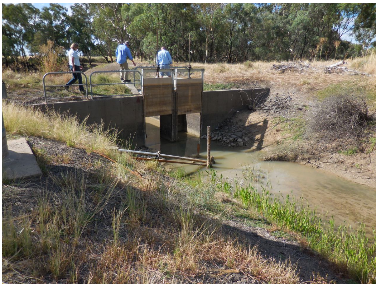
Figure 4. Finley Escape at the junction with Billabong Creek
